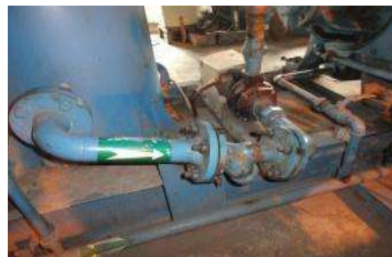
Fig. 10 Recirculation pump in vacuum system
