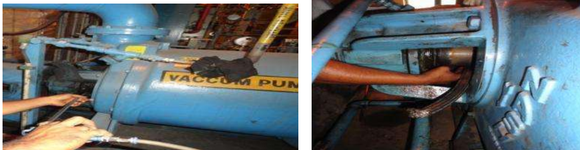
Fig.7 Wear Gland packing replaced by one gland packing
