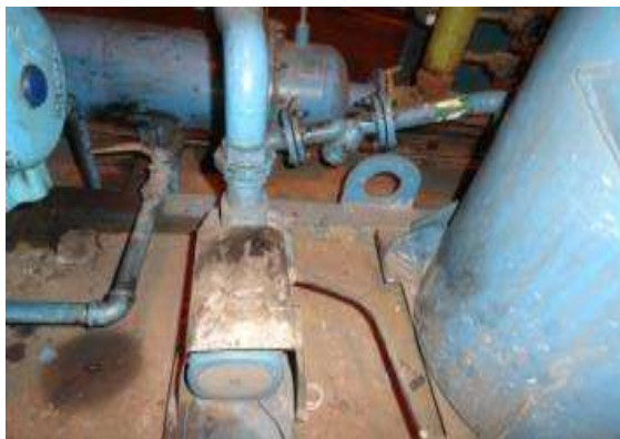
Fig. 10 Recirculation pump in vacuum system
