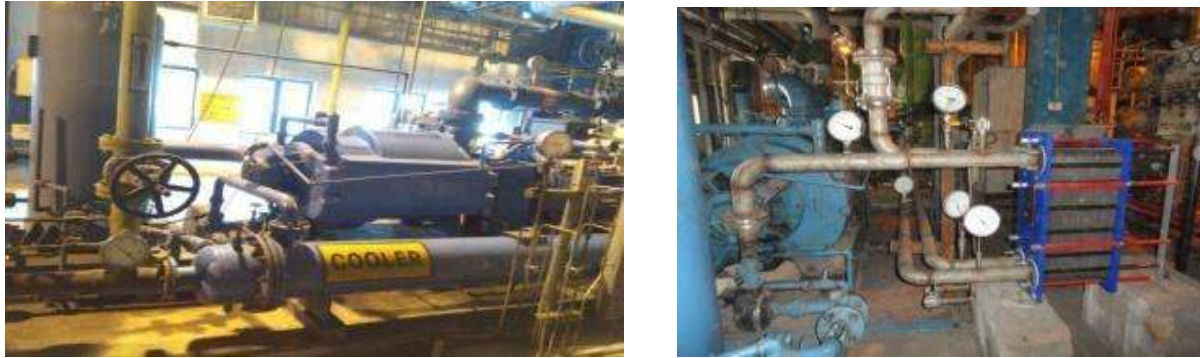
Fig. 6 Replacements of existing shell and tube cooler by plate type heat exchanger
