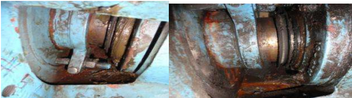
Fig. 16 Vacuum pumps bearing excess lubrication
