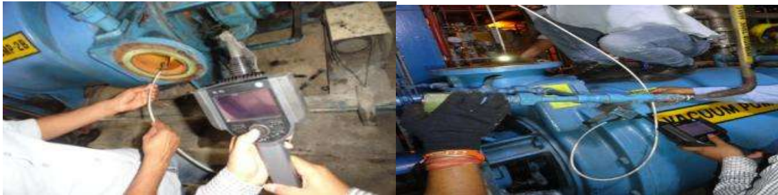
Fig.11 Boroscope inspections of second stage and first stage of Vacuum pump rotor.
