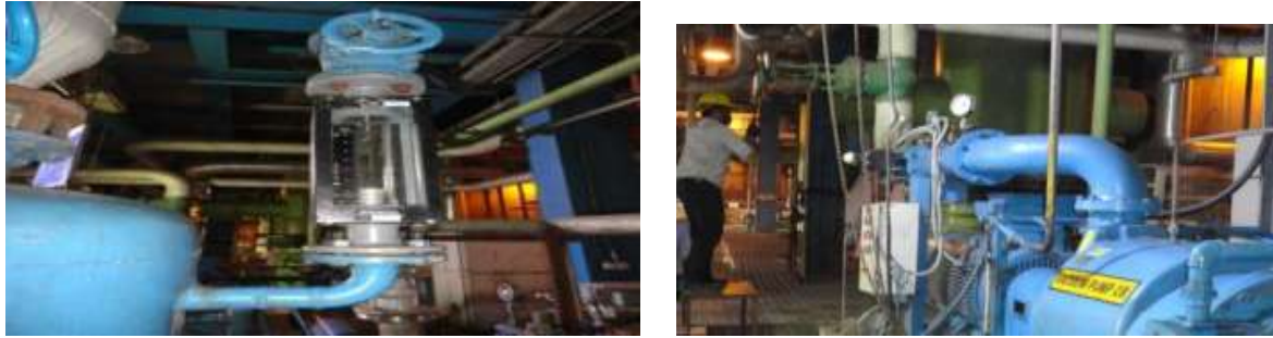
Fig. 4 Air ingress in rotameter during shut off head
