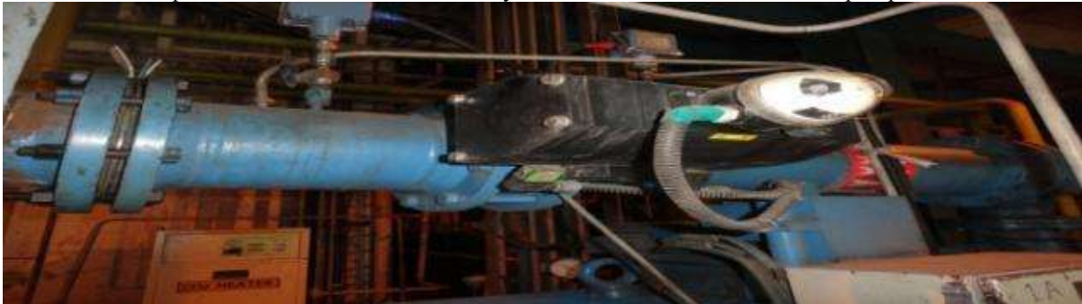
Fig. 18 Suction butterfly valve
