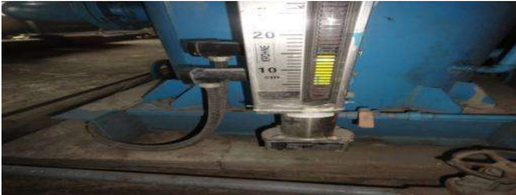
Fig. 9 Normal water levels in separator tank
