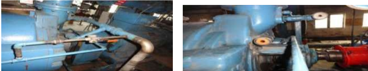
Fig. 2 Sealing water spray nozzle and replacement of gland sealing line valve.
