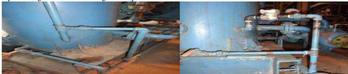
Fig. 22 Recommendations for NRV installation overflow loop NRV missing
