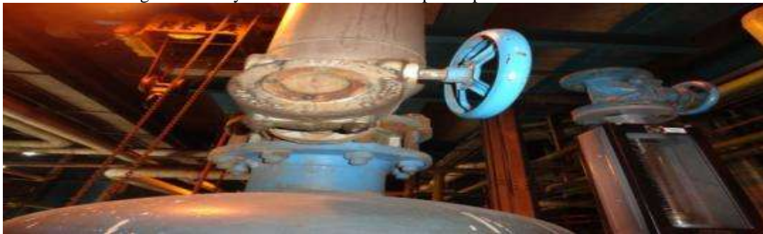
Fig. 17 Manual butterfly valve on separator tank
